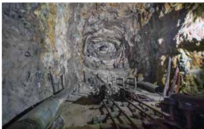
An impressive display at Rzeczka, in one of the massive cross passages. The scale can be judged by the human mannequins at work on the clear working platform or benches. Photo Chris Rayner
